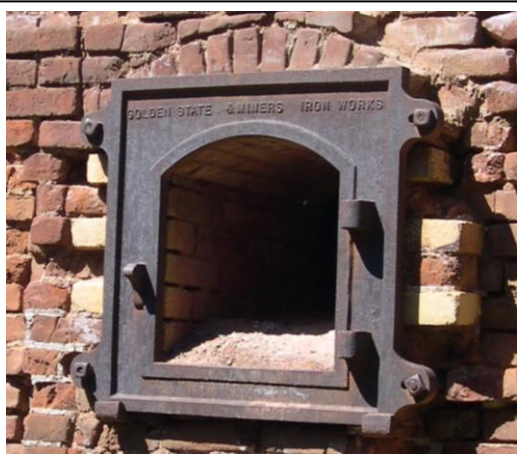
Figure 7. Close-up of one of the furnace's ovens, imprinted with the name of the manufacturer: "Golden State & Miners Iron Works."
