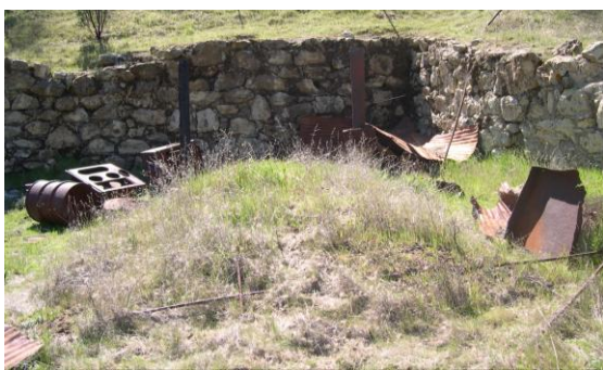
Figure 15. Grassy mound in the middle of structure 1. Several pipes found around edge of mound, but no clues on the surface about what might be inside.
