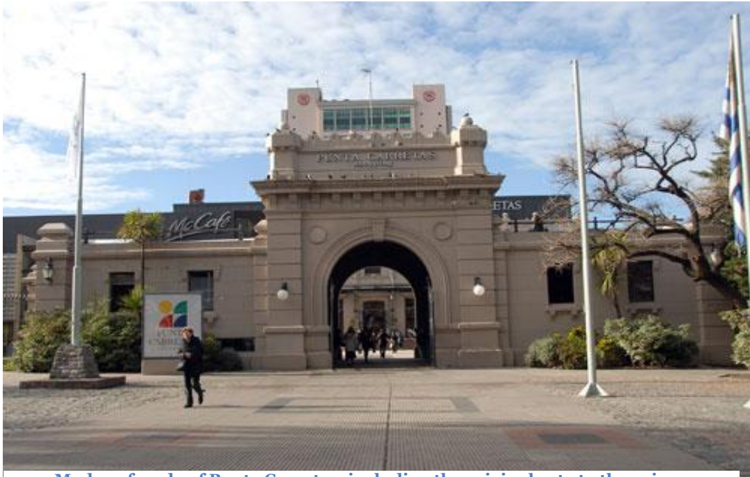
Modern façade of Punta Carretas, including the original gate to the prison
