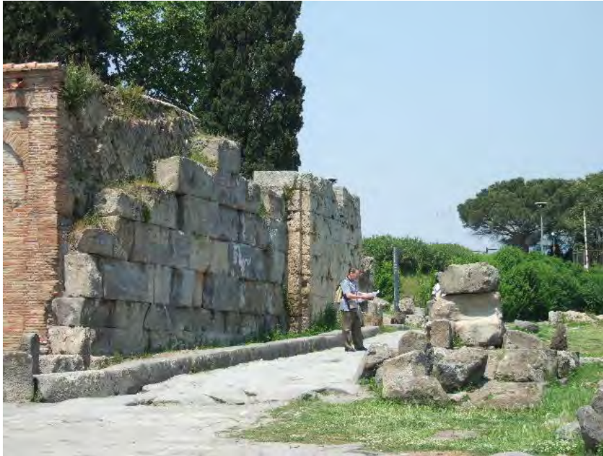
Fig. 2 – Example of opus quadratum
