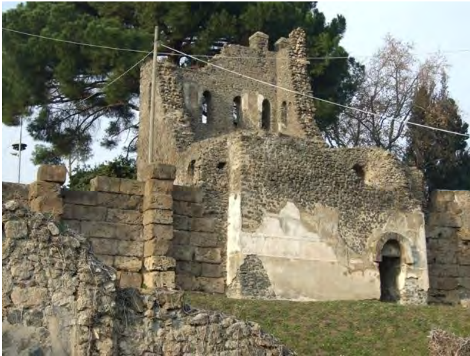
Fig 6. – Tower construction materials, opus incertum , plaster visible at base with relief imitating surrounding opus quadratum wall.
