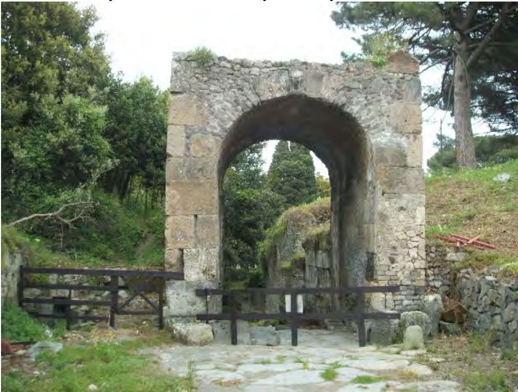
Fig. 4 – Refurbishment of gate in opus incertum , visible at top
